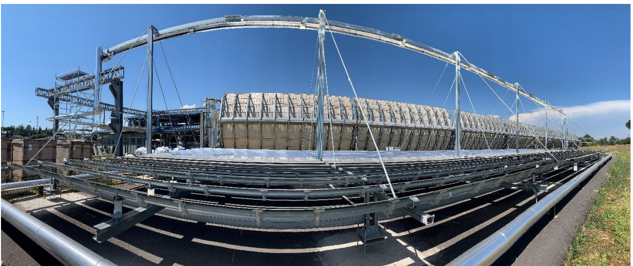
Figure 24: Visit to ENEA Casaccia research centre - linear fresnel and parabolic trough (back)
